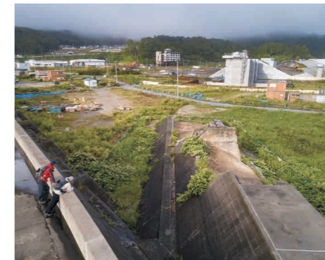
The Tarocho breakwater and hotel destroyed by the tsunami, and the new storm surge barrier
